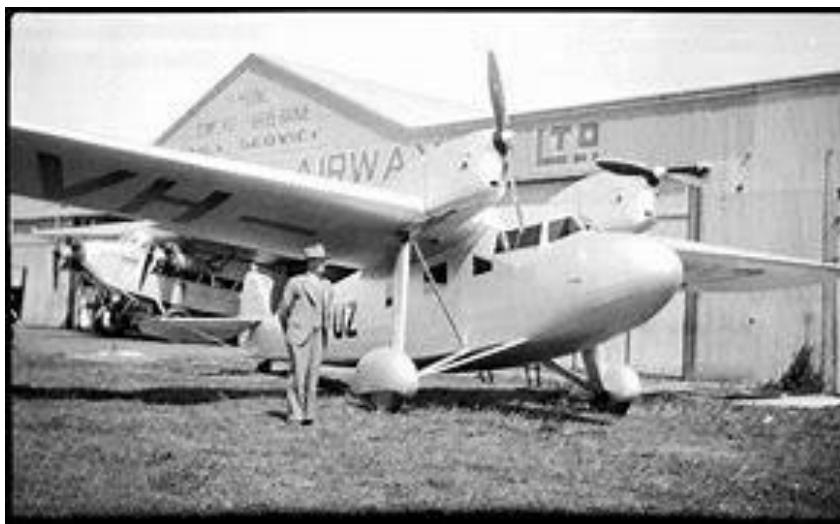
The Codock's construction was a welded metal fuselage frame and tailplane unit, covered with fabric, whereas the wing was a wooden cantilevered structure. The cockpit accommodated two pilots, and the cabin could carry up to six passengers or 762 kg of freight. Provision could be made for two stretcher patients and a nurse.
